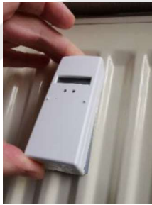
6-10 MOUNTING EHCA ON HEAT CONDUCTOR
